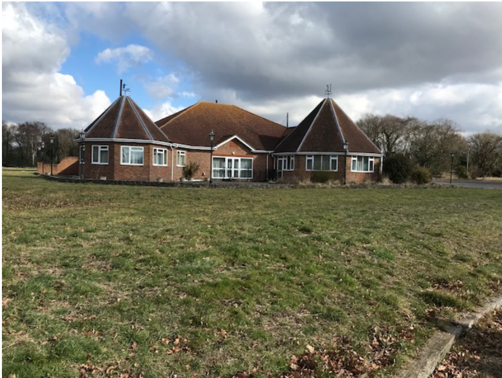
Existing building and hardstanding inside the site
